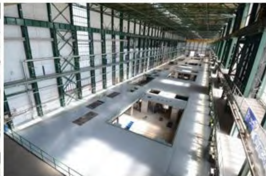
Turbine hall after dismantling (11/2016)
