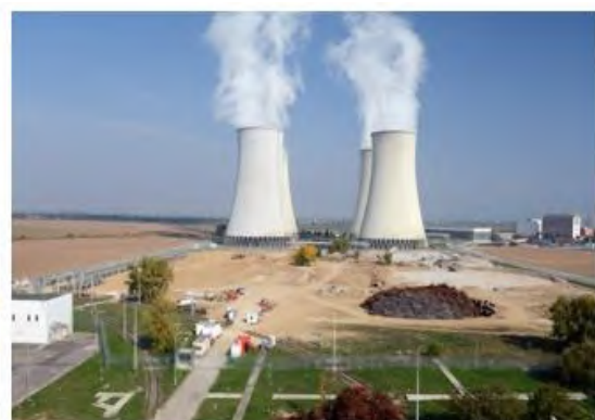
After demolition of 4 cooling towers (10/2018)
