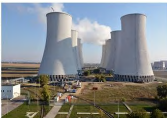
Before demolition of 4 cooling towers (09/2017)
